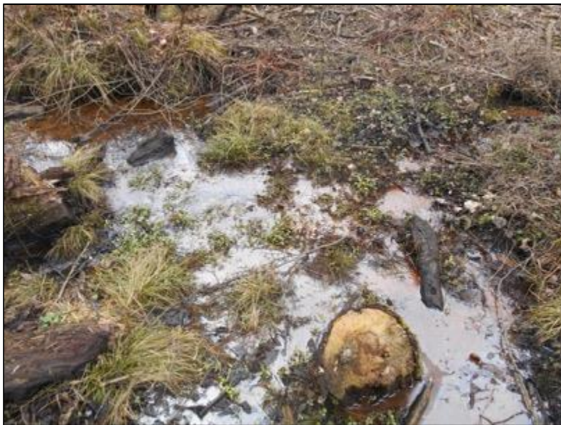
Downstream toe area – no drainage due to absence of gradient away from dam toe.
