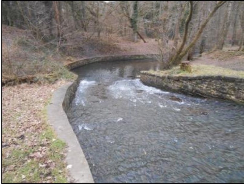
Spillway channel.
